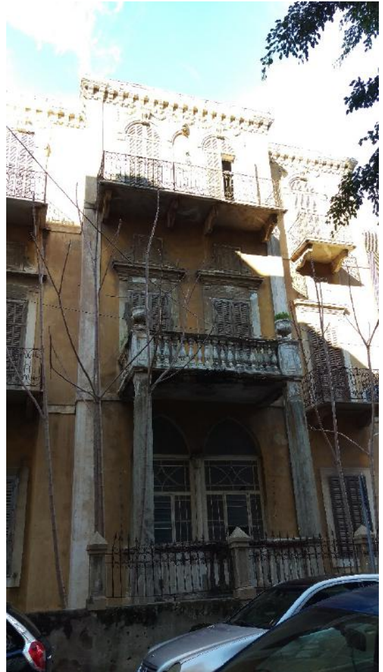
Figure 27: Abandoned mandate building with a classical central bay and veranda on Saint Joseph street
