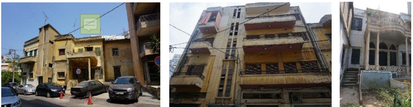
Figure 51: Different abandoned buildings
