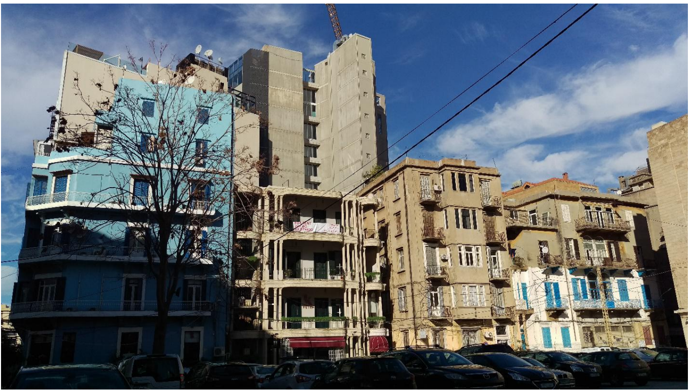
Figure 22 21: Four typical typologies aligned on Saint Joseph street (Yessouiyeh): from left to right, 1950s building (modern), veranda-type building (intermediate transitional), Building with bay-windows (late transitional and building with central bay / double arcade (Intermediate transitional)
